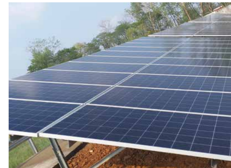
Installation of Solar Power Panels: A push for Renewable Energy
