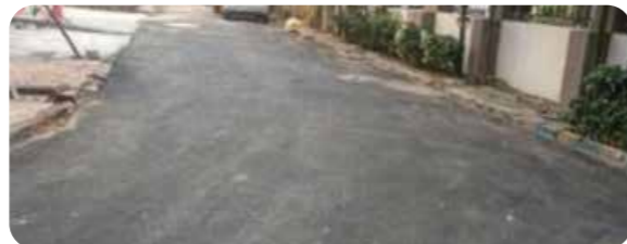
Waste plastic road works at ERO
