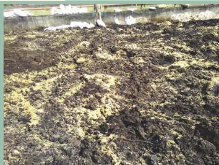
Bio-remediation at Oil soaked soil at Chainage
