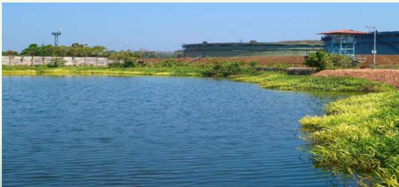
Rain water harvesting at Kochi Refinery
